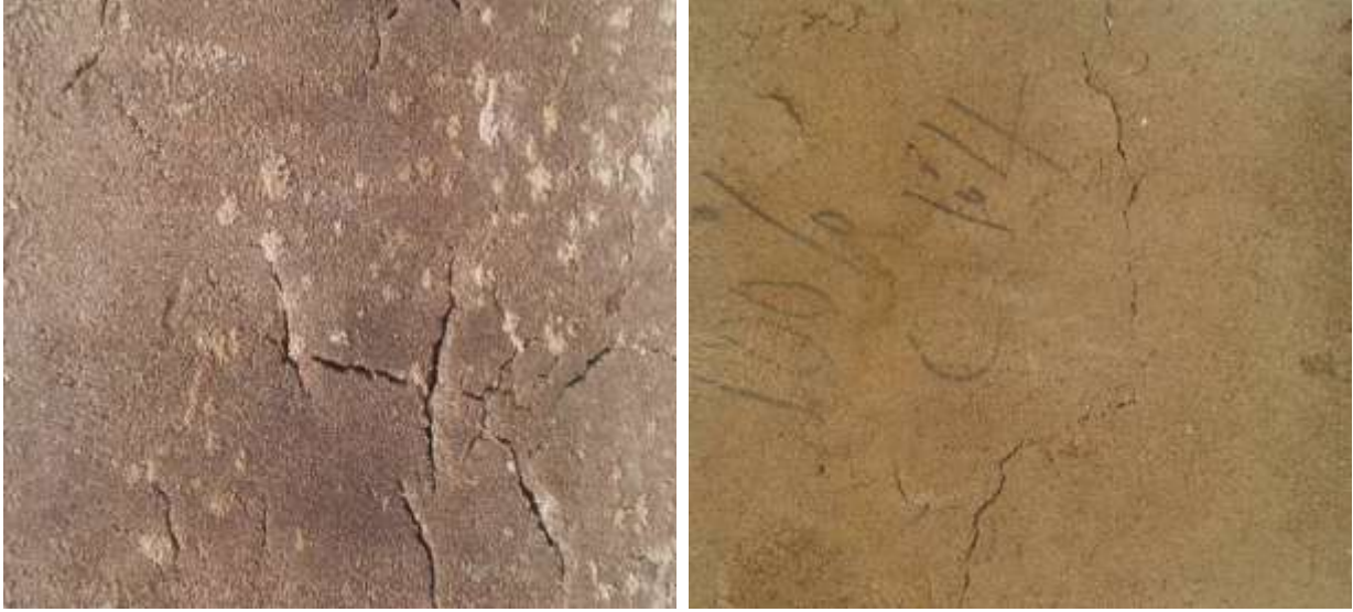
Plate 1: Showing walls plastered with local brewery waste and bitter cassava flour and sand
