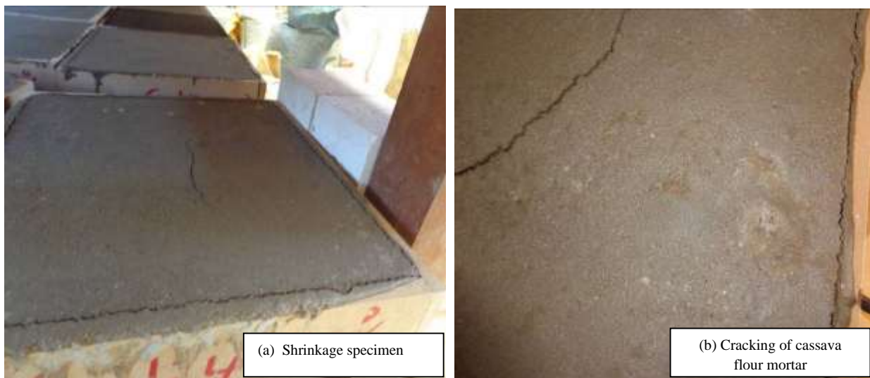
Plate 4.2: The cracking of cassava flour and cement blended mortar
