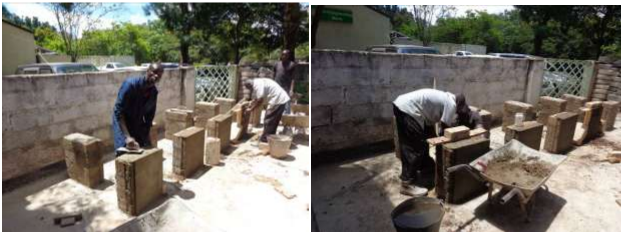
Plate 3.3: The walls being plastered with different mortar mix
