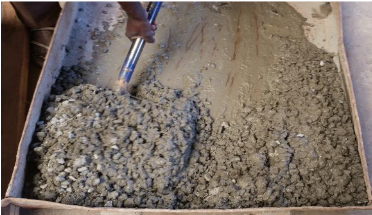
Figure 3.4: Mixing of concrete to obtain a homogenous mix
