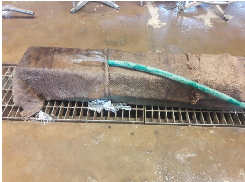
. Plates 3.7: Curing process of beams under membranes.
