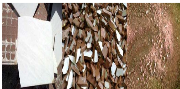
Figure 1: Ceramicclay tile waste at demolition site
