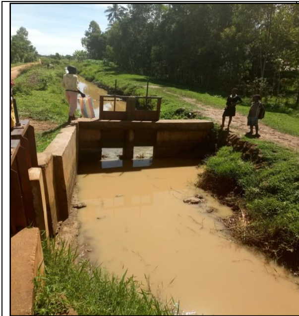
(a) Gate in Bunyala irrigation scheme
