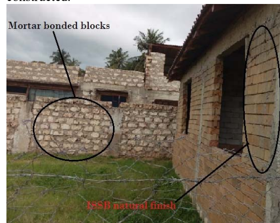
(a) Wall appearance of mortar bonded blocks and ISSB
